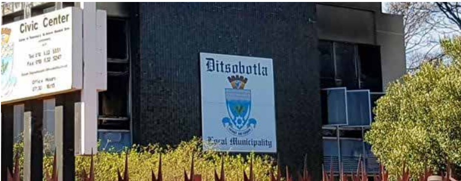
Ditsobotla Local Municipality. Picture: Supplied
