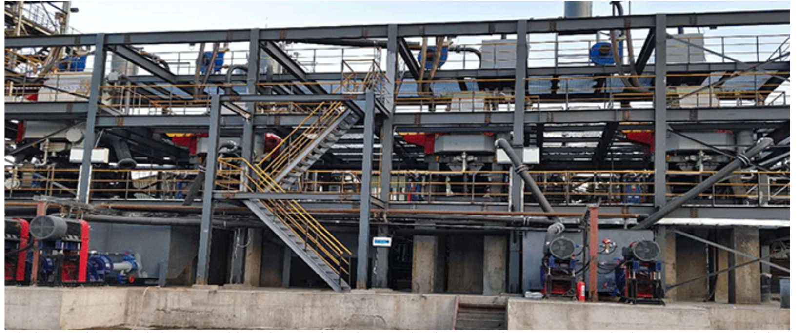
A shocking 43% of chrome wash plants inspected during the current financial year were found operating without any environmental authorisations. Pictures: Supplied
