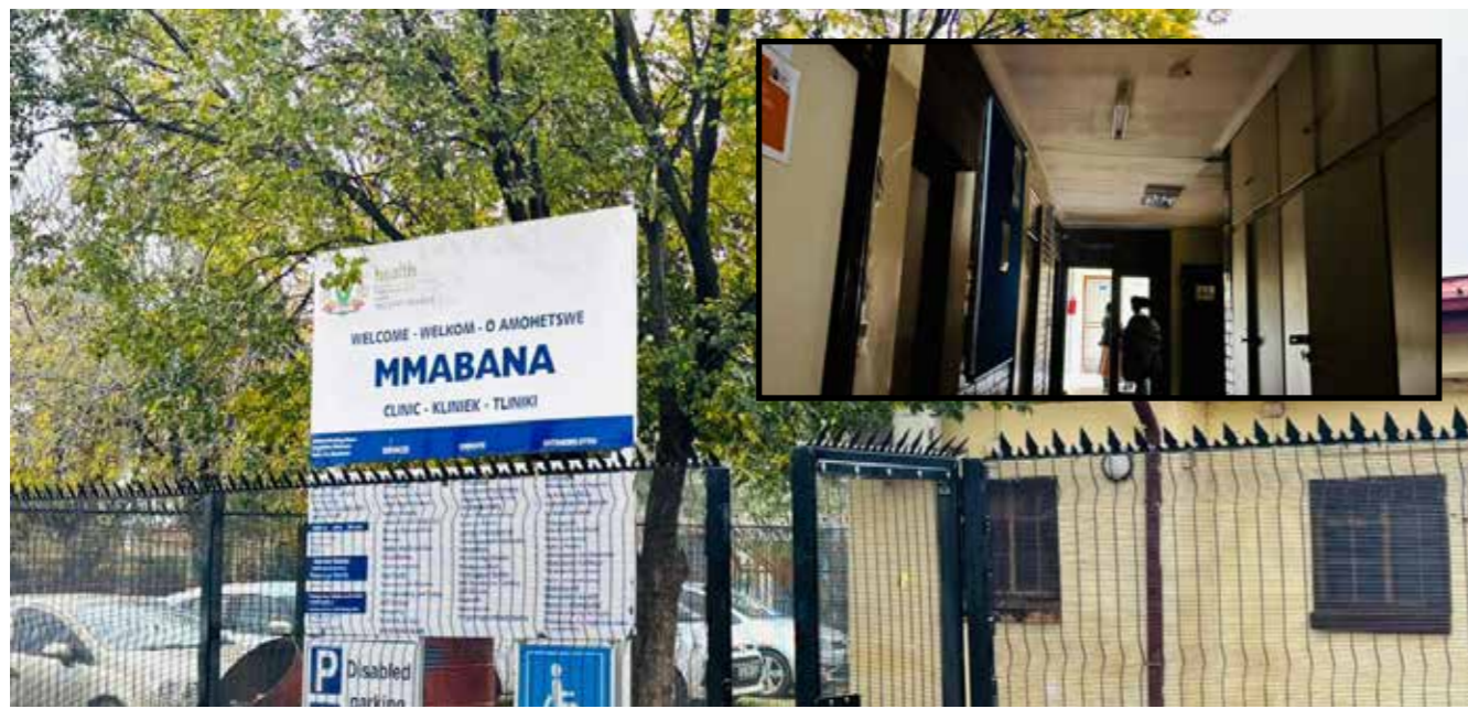
Mmabana local clinic in the second month without electricity. Picture: Thembisile Mlangeni
