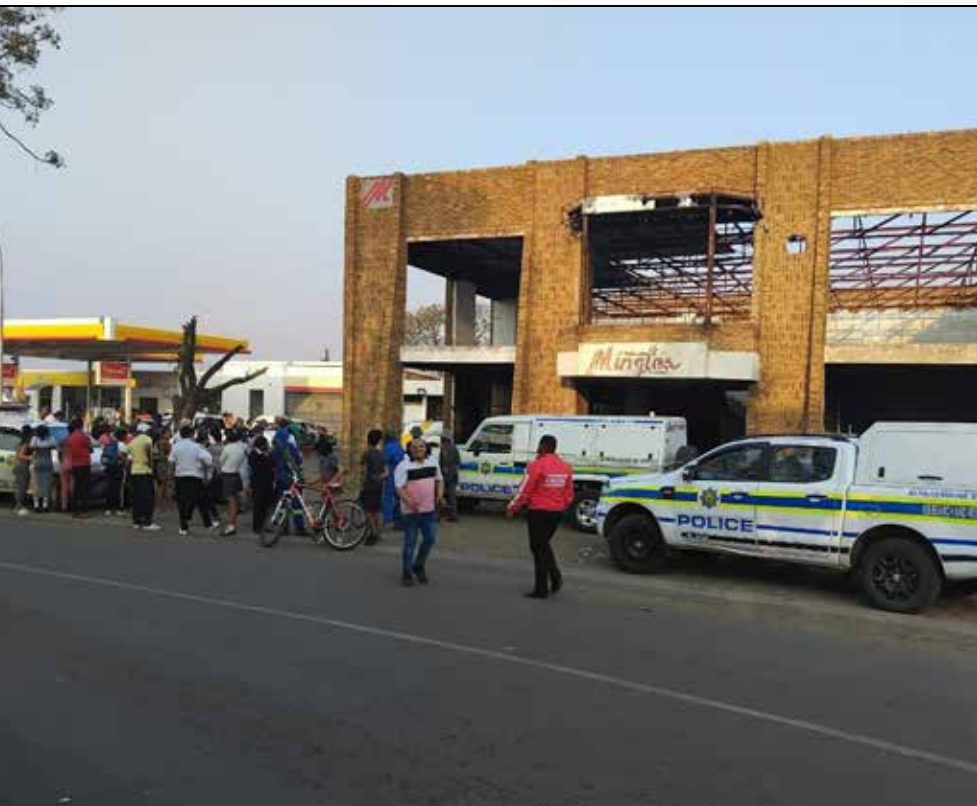
A decomposed female torso and legs found floating in the flooded basement of a dilapidated nightclub in Heidedal. Picture: Supplied
