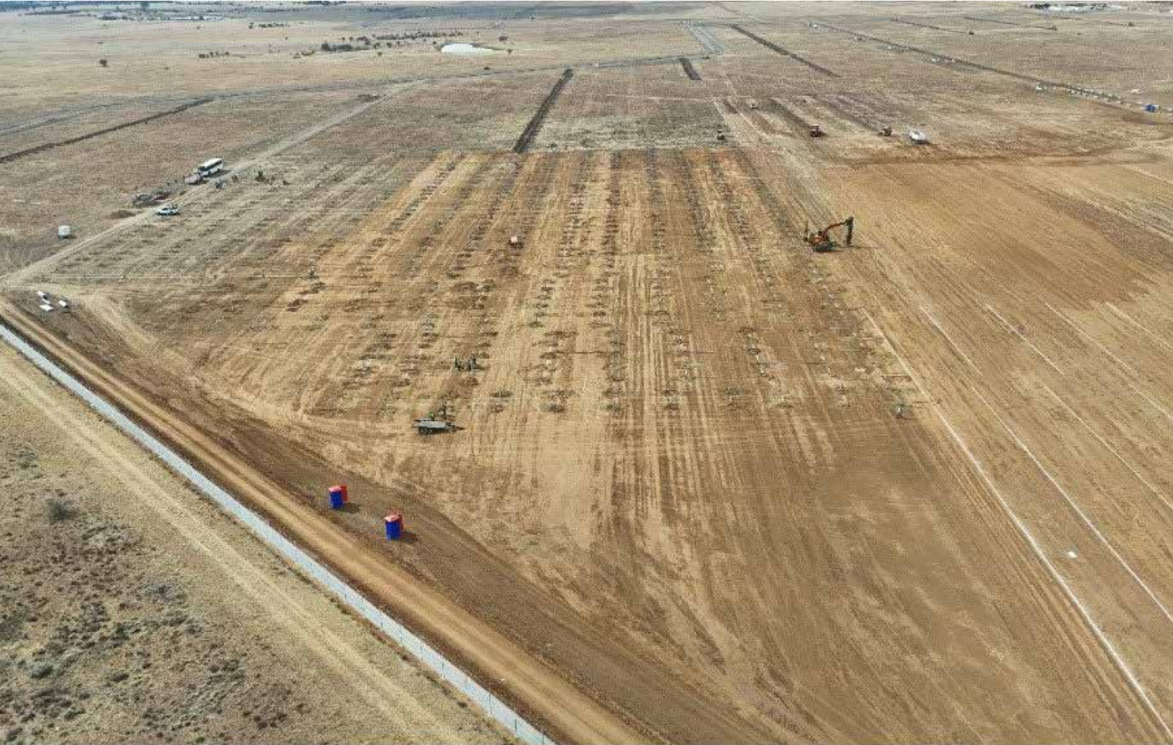
157 MW Khauta West solar PV facility under construction. Picture: Supplied
