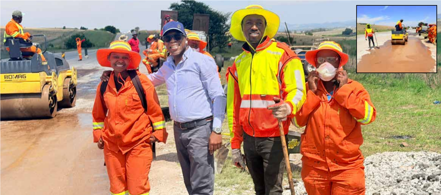
Ngwathe Local Municipality Municipal Manager Dr. Futhuli Mothamaha during his site inspection on Tuesday, engaging directly with repair teams, assessing progress, and reinforcing the need to address road hazards without unnecessary delays. Photo: Supplied
